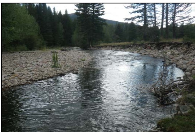
Photo 17. Eroding bank Tenderfoot Creek (AQ5), looking downstream aspect.
